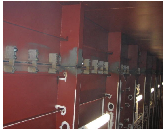
Plate fairing inside hull
