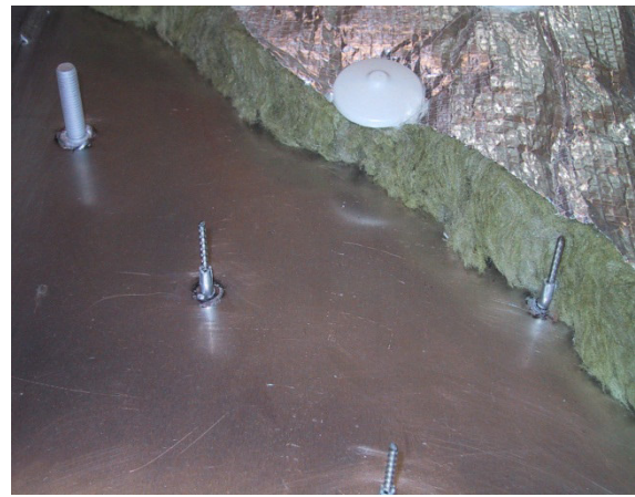
Pin type VBS + clip type WN
