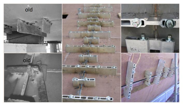
Hilbig high speed fastening systems for deck plate fairing using aluminium bridges
